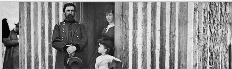
[Detail] City Point, Va. Brig. Gen. John A. Rawlins...
